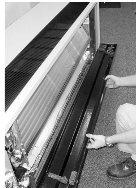
Figure 52: Slide drain pan out of unit for inspection/cleaning.
