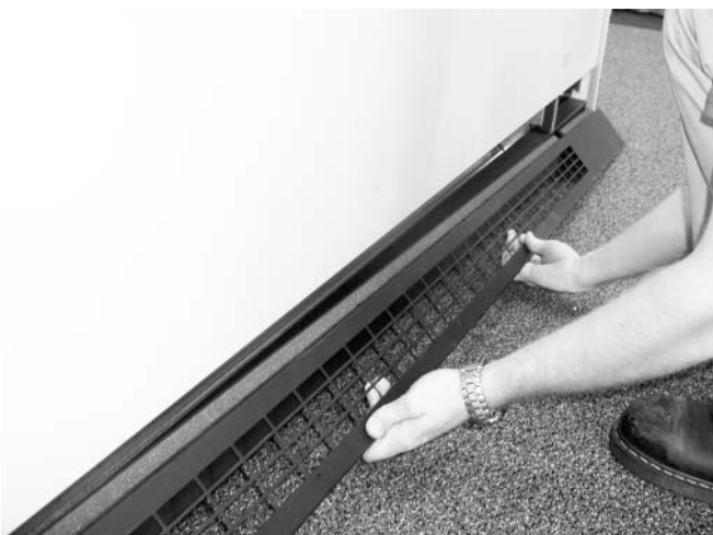
Figure 48: For filter replacement, remove the screws holding the front air grille and remove the grille.
