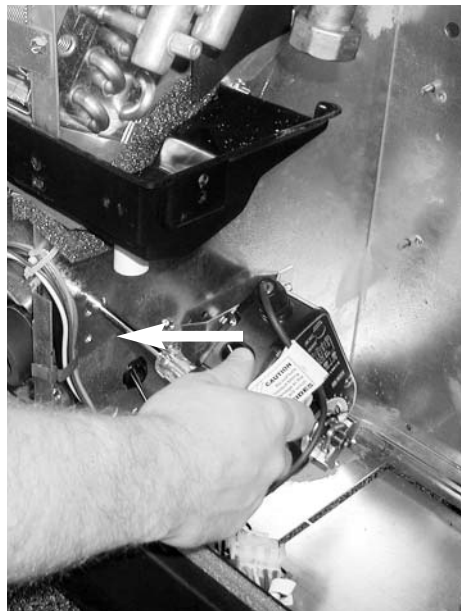
Figure 50: Removal of screws in support plate of drain pan.
