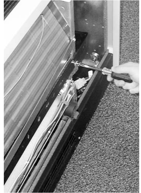
Figure 51: Removal of screws holding drain pan in place.
