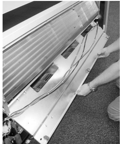
Figure 54: Slide fan board forward to remove.
