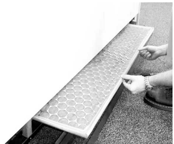
Figure 49: Slide out old filter and replace with new filter. Reattach return air grille.
